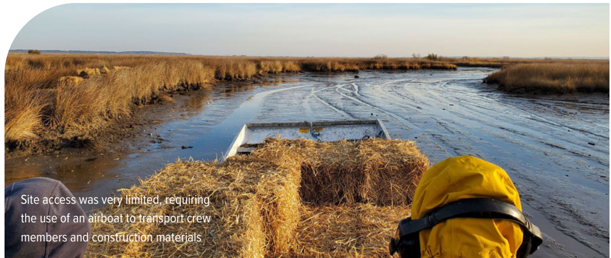
Lower Wicomico Dredging and thin layer placement marsh enhancement. Straw bale dike.
