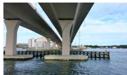
Typical 10-pile channel pier elevation shown at Pier 4
