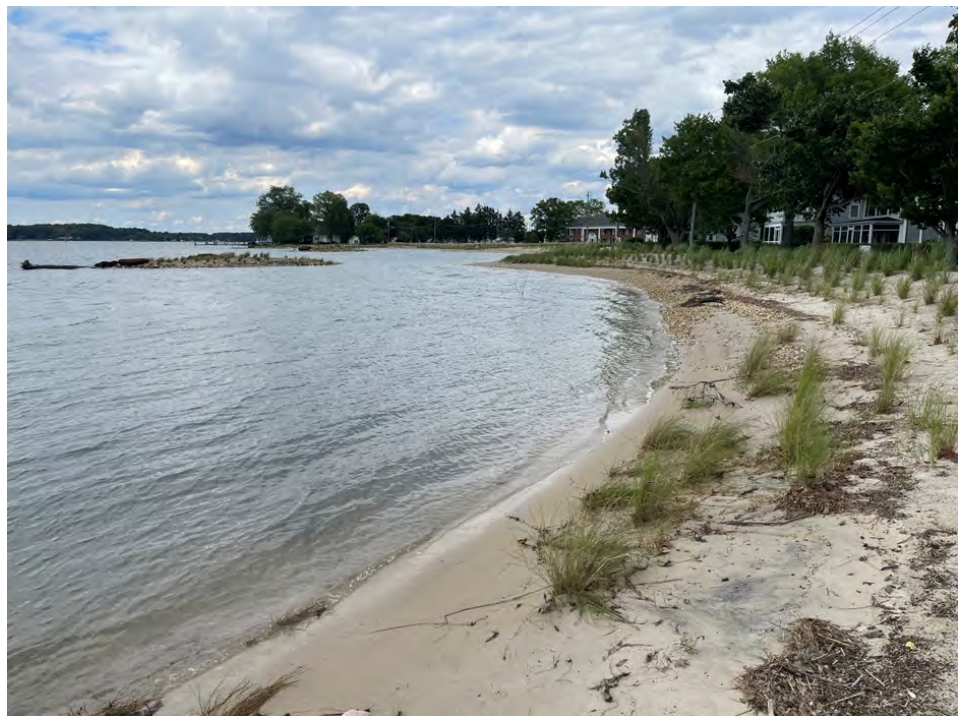
Photo 4 | Beach and Dune Creation as part of a Living Breakwater project on the Tred Avon River in Oxford, MD. The project, designed by team member Keith Binsted, included offshore living breakwaters and marsh, beach, and dune creation to increase coastal resiliency of low-lying roads and homes.
