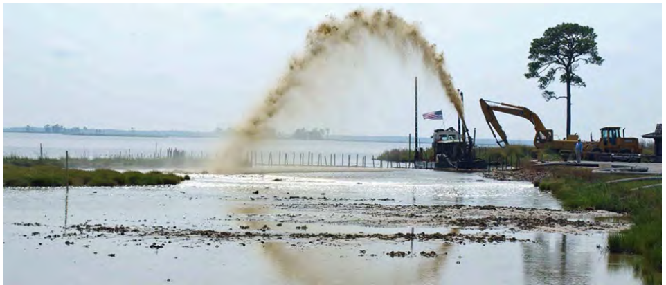
Photo 5 | Thin Layer Placement (TLP) has been successfully implemented in the Chesapeake Bay to enhance tidal marsh elevation and resilience in response to subsidence, sea level rise, and erosion. Projects such as the Blackwater National Wildlife Refuge restoration demonstrate that carefully controlled sediment placement can raise marsh elevations while allowing vegetation to persist and recover, supporting long term marsh function and ecosystem stability. Image source: U.S. Army Corps of Engineers, ERDC - https://tlp.el.erdc.dren.mil/
