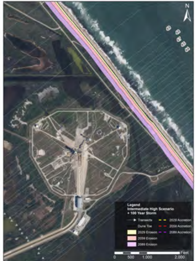
Illustration of Atlantic Shoreline Near Launch Infrastructure Showing Increased Level of Erosion Risk as SLR Increases for 2029 (Yellow), 2059 (Red), and 2089 (Purple).
