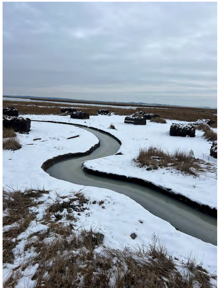
Photo 6 | Constructed runnel and high marsh hummocks at Langmaid Salt Marsh Restoration, designed by Straughan Environmental
