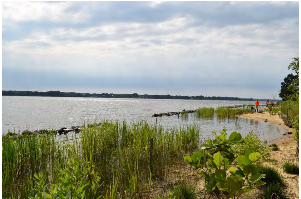
Photo 3 | Cedar Haven Living Shoreline on the Patuxent River. Designed by Straughan Environmental, this project included installation of a stone sill, sand nourishment, and bank grading to improve coastal resilience and provide habitat for estuarine species.
