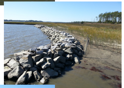
Captain Sinclair Marsh Sill Post Construction
