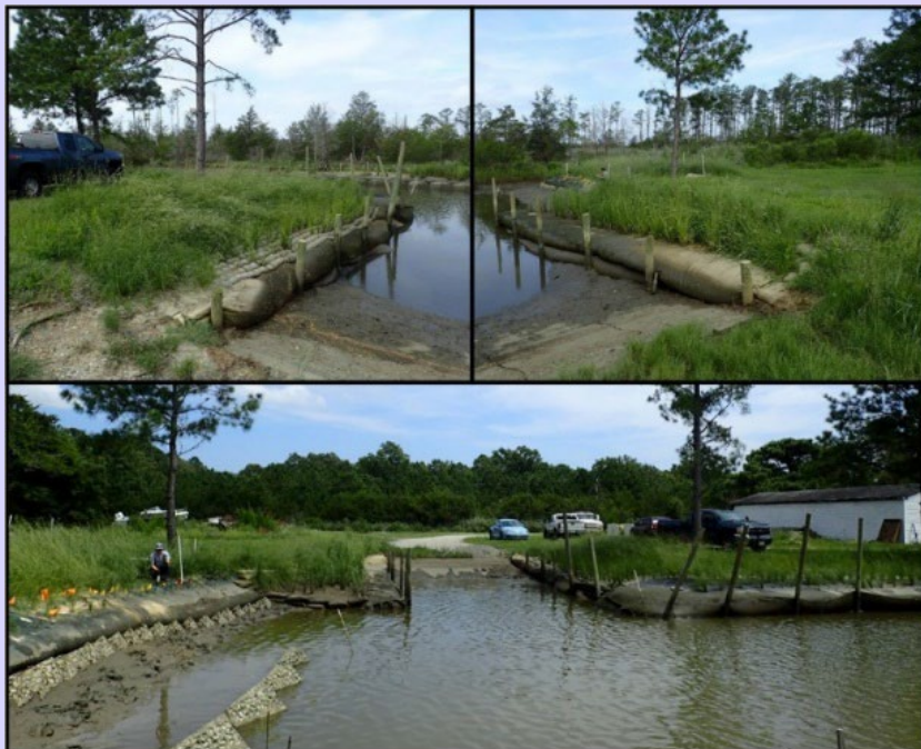
Figure 24: Whittaker Creek Shoreline Protection Project seen with lush marsh grasses thriving months after project completion in 2024 at this Middle Peninsula Chesapeake Bay Public Access Authority Property - Captain Sinclair's
