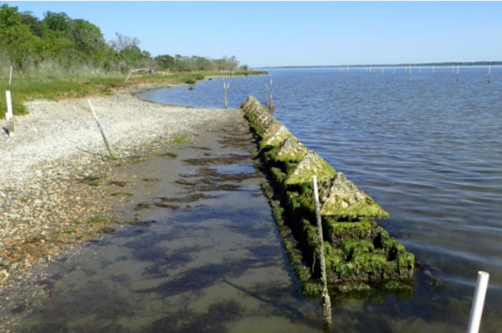
Figure 15: Living shoreline reef with Castle Toppers constructed at the NWSY Summer 2024 by Getting It Done Co. A tombolo of sand can be seen forming in the lee of the structure after 1 year.
