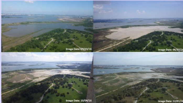
Figure 27: Aerial view before and after for Barbours Cut Dock Expansion and San Jacinto Marsh Restoration Project
