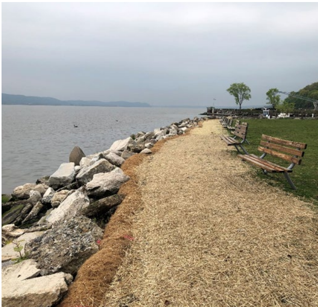
Figure 11: In a design by Doug Gaffney, coir logs were used to restore the Hudson River shoreline of a waterfront park affected by SLR and winter storms. Rapid response was facilitated by an understanding of permit rules (2023).
