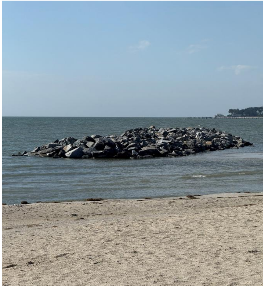
Photograph of offshore breakwater built with rocks. Image Credit: Laura J. Whitaker.
