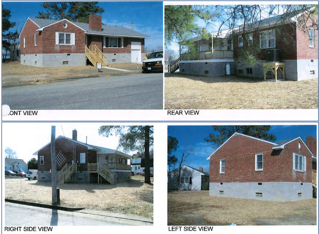
Figure 153: Photos of a home in the Town of West Point after being elevated.
