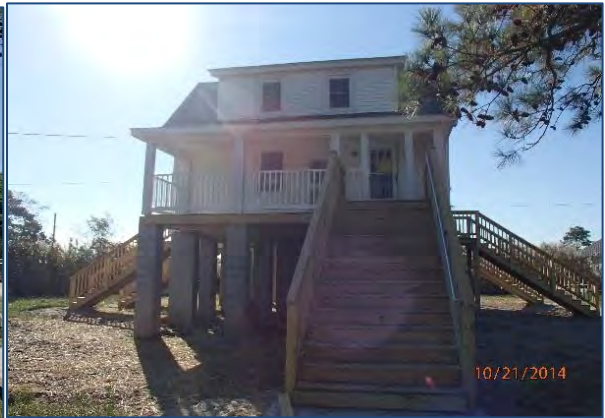
Figure 145: House in Hayes, Gloucester County - AFTER elevation.
