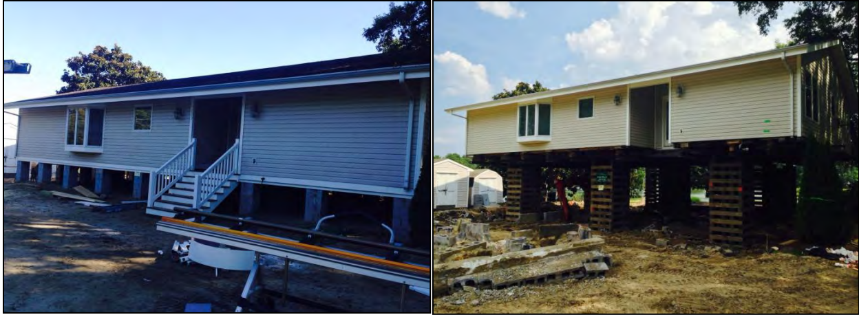
Figure 122: Photos of an elevated home in Port Haywood during (left) and after (right) being elevated (Mathews County, 2015).
