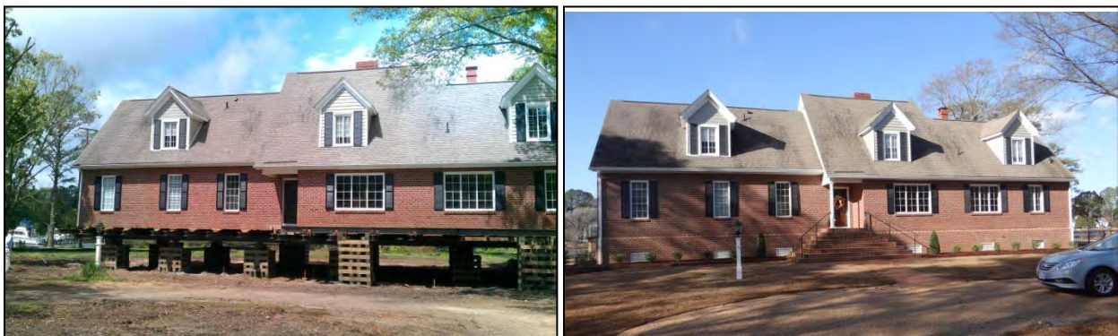
Figure 150: Photos of an elevated home in Moon, Va during (left) and after (right) (Mathews County, 2015).
