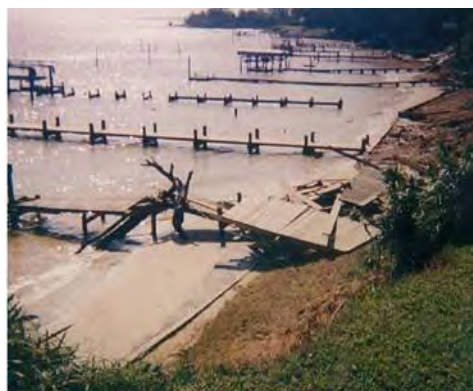
Storm damage incurred on the York River during Hurricane Isabel, 2003. Photo credit: J. Rickards.
