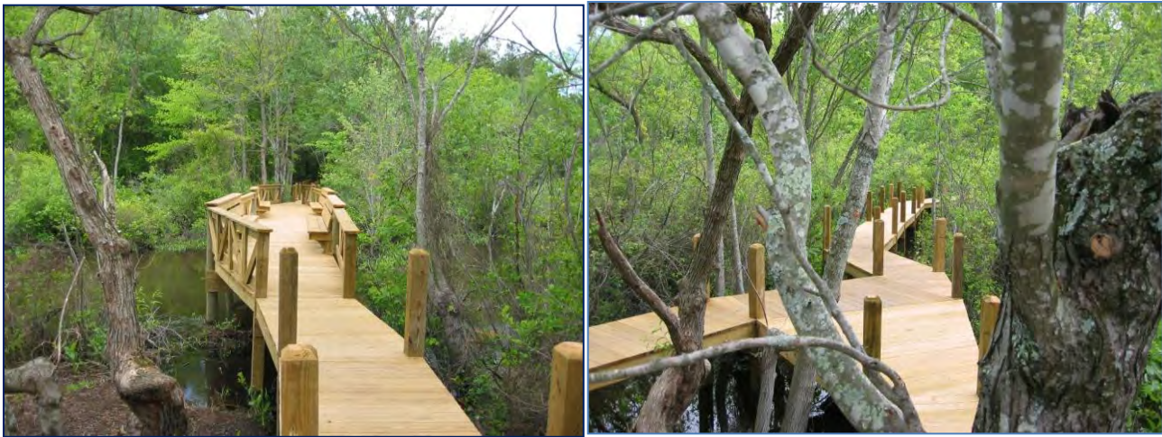
Figure 14: Photos of the bridge across the Dragon Run (below).
