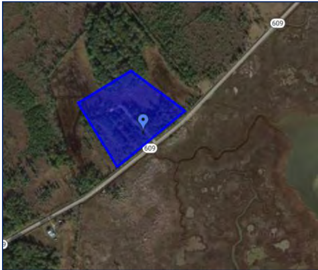
Figure 25: Aerial of Winter Harbor North.
