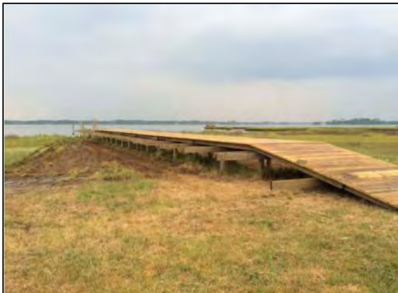
Figure 7: Newly constructed public access pier.
